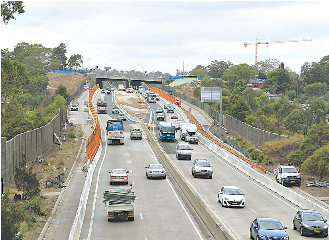
Windsor Road west facing ramps.
